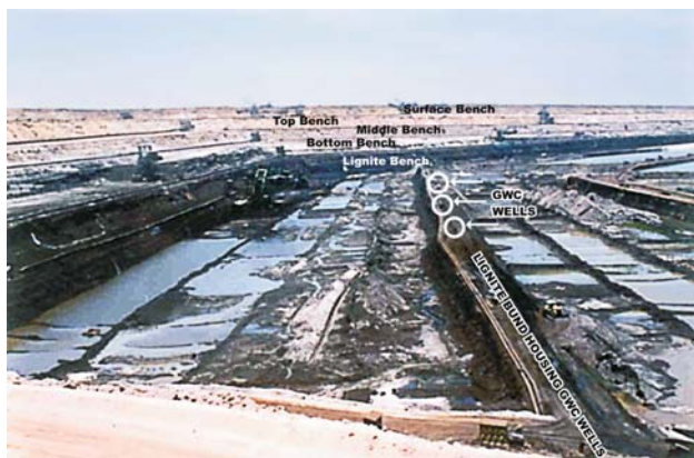
Fig. 5 Depressurisation strategy adopted in the Neyveli lignite mines (Source: Gowrishankaran 1980)
